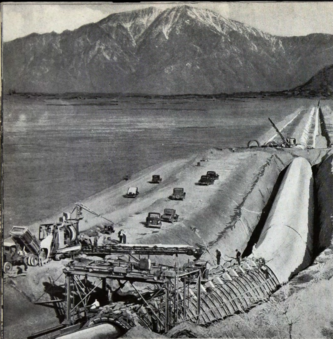
On the way! Section of Aqueduct conduit under construction west of San Jacinto Mt.
