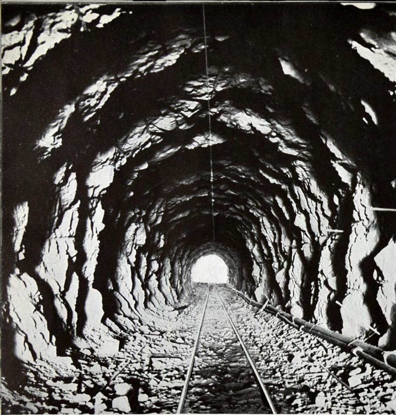
Typical Aqueduct hard rock tunnel, 18 feet in diameter before being lined with concrete.
