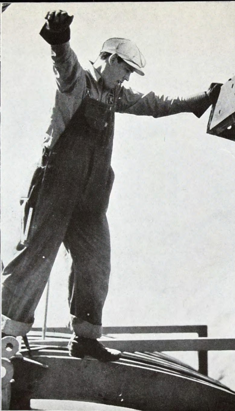
Steel form workman on Aqueduct conduit section.
