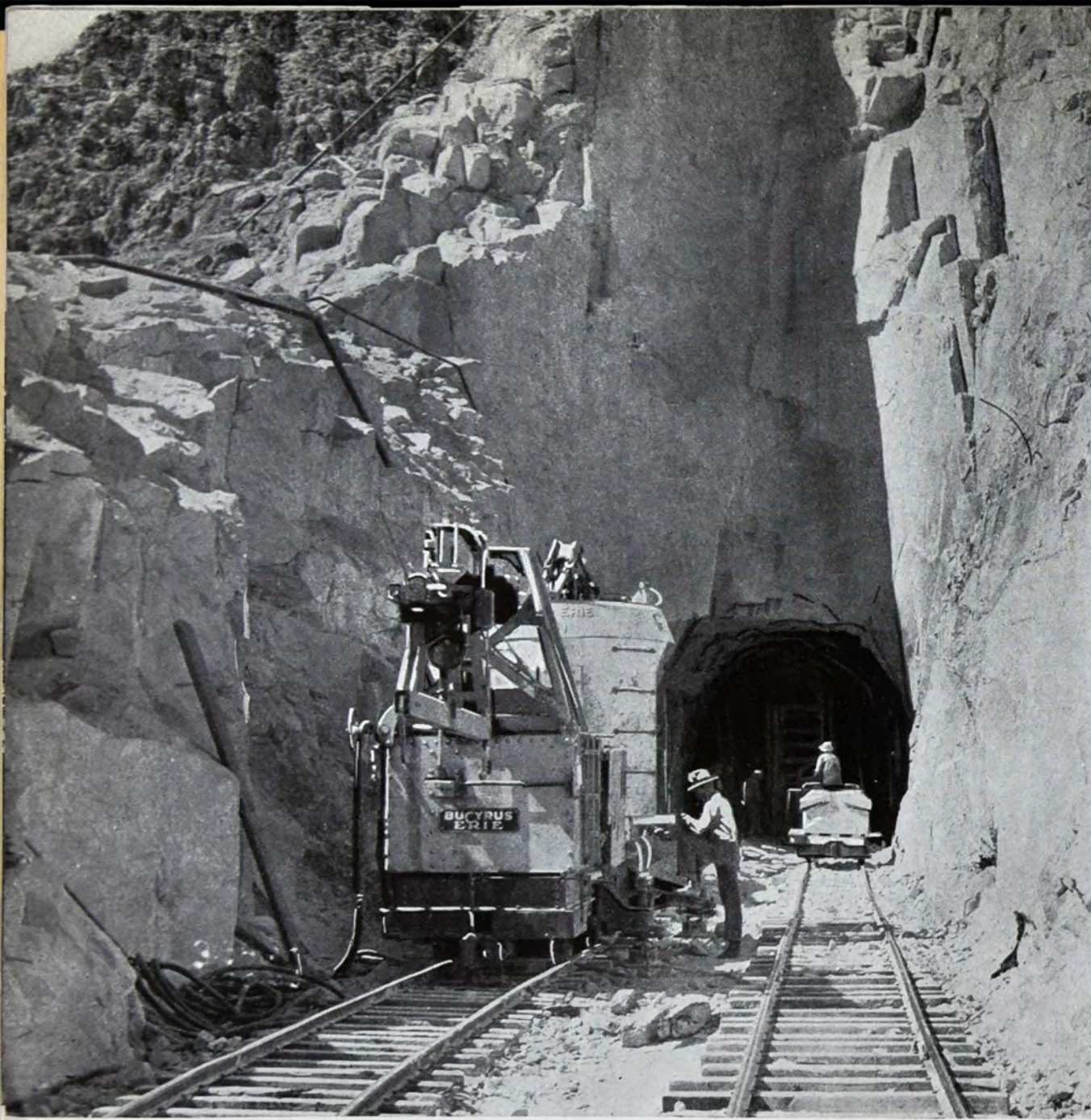
East Portal, Coxcomb tunnel, one of 29 hard rock tunnels totaling 92 miles in length on Aqueduct main line.
