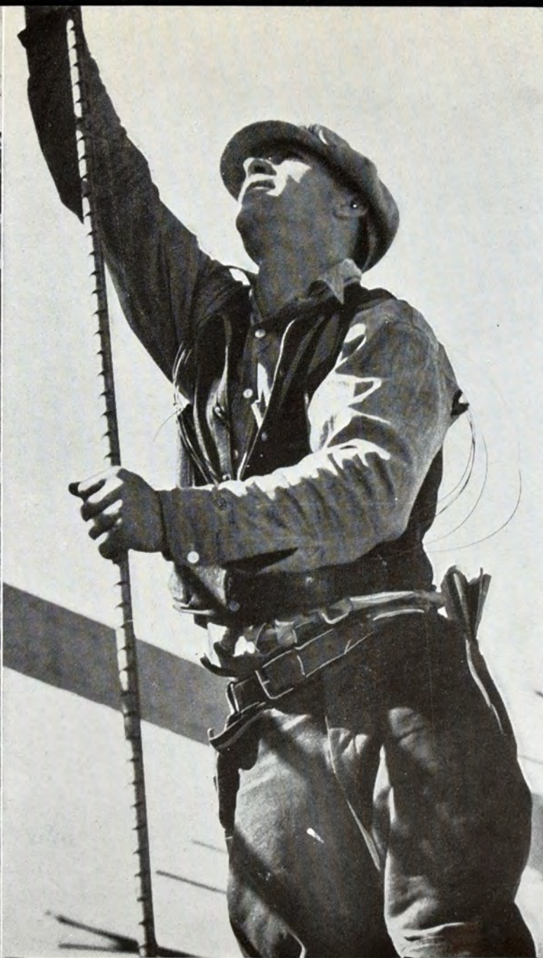
Reinforcing steel workman on an Aqueduct siphon section.
