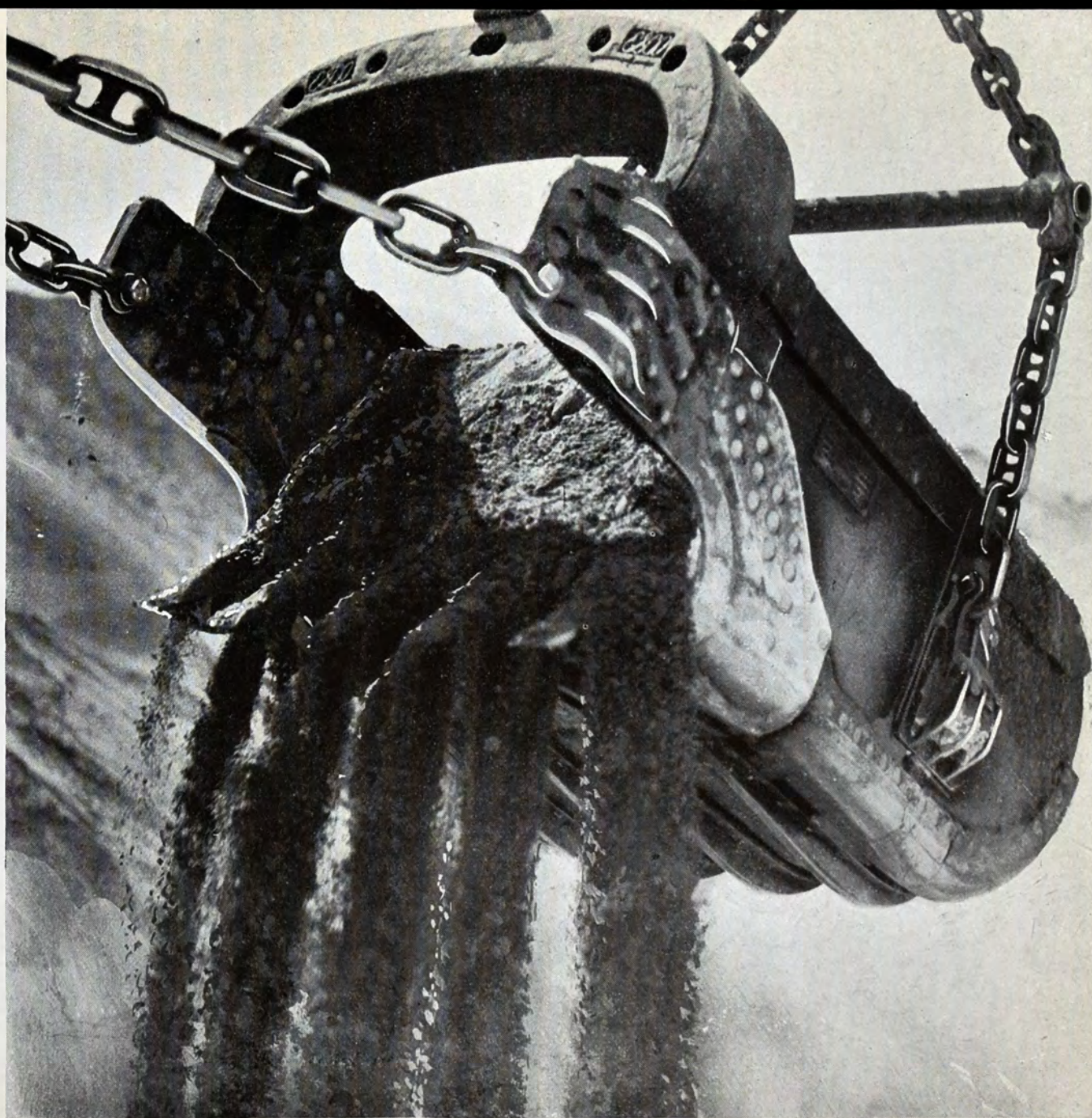
On the Big Job! A shovelful of the 45,000,000 cubic yards of Aqueduct material being excavated.
