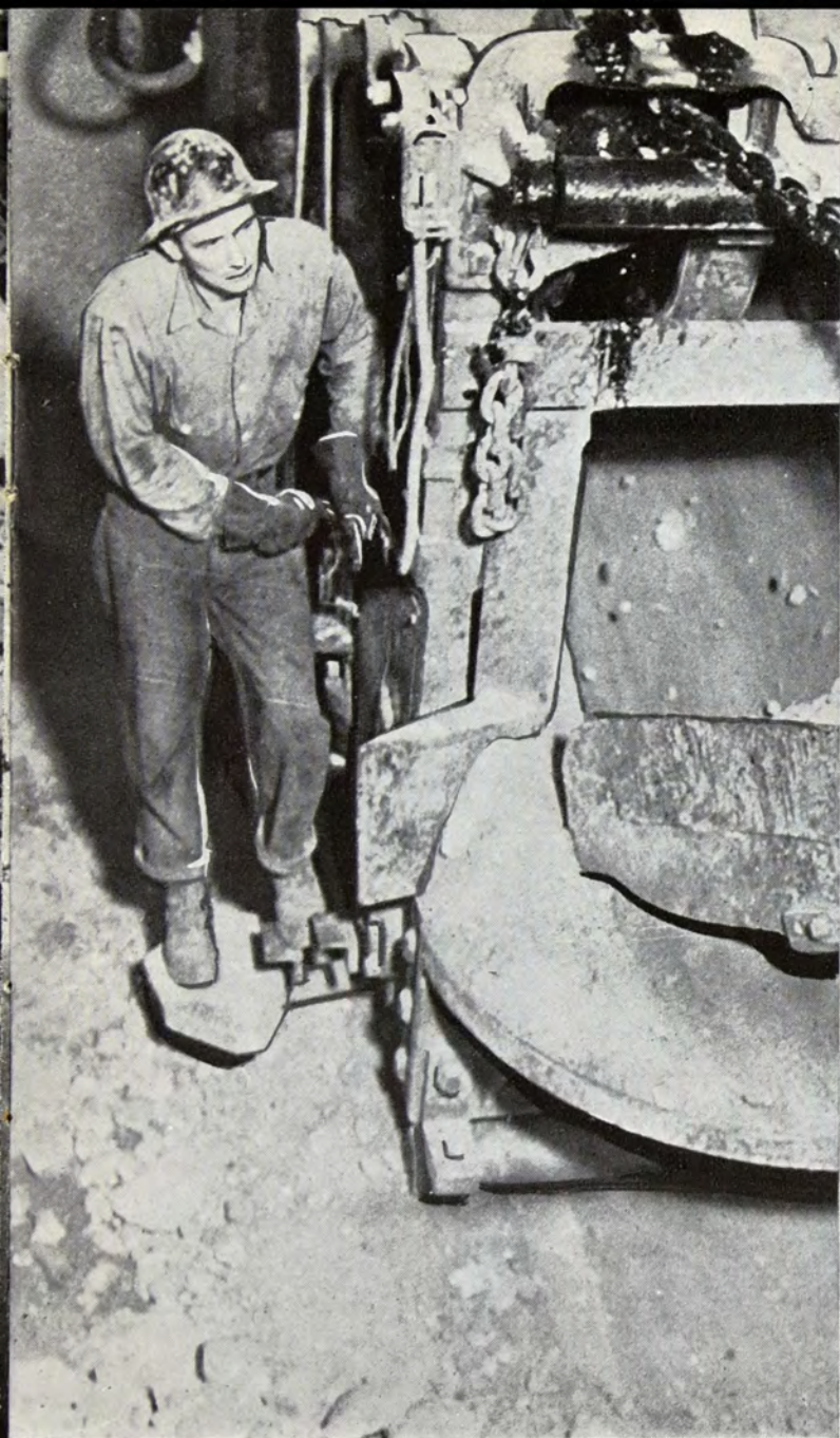
Mucking machine operator in an Aqueduct tunnel.
