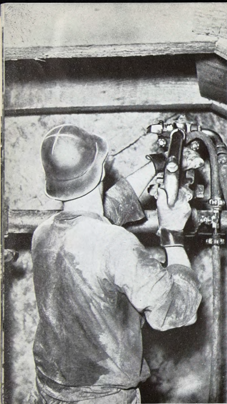
Drill runner in a hard rock Aqueduct tunnel.
