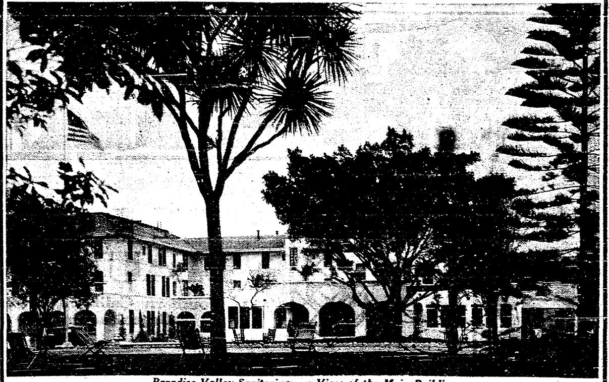
Paradise Valley Sanitarium—a View of the Main Building
