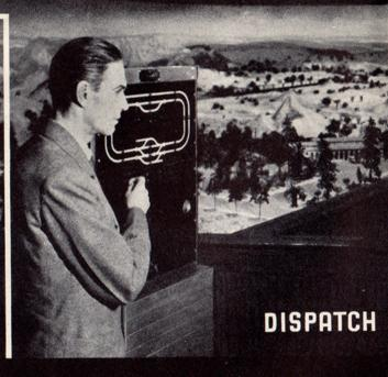
from a central dispatch board, so connected with the automatic signals that it is impossible to make an error that will cause an accident
