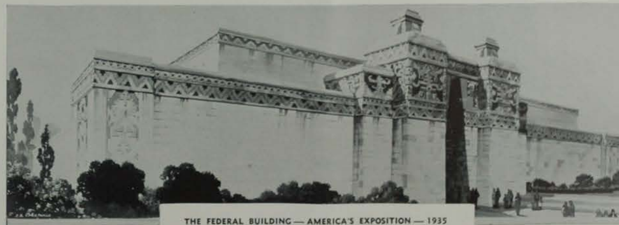
THE FEDERAL BUILDING — AMERICA'S EXPOSITION — 1935
