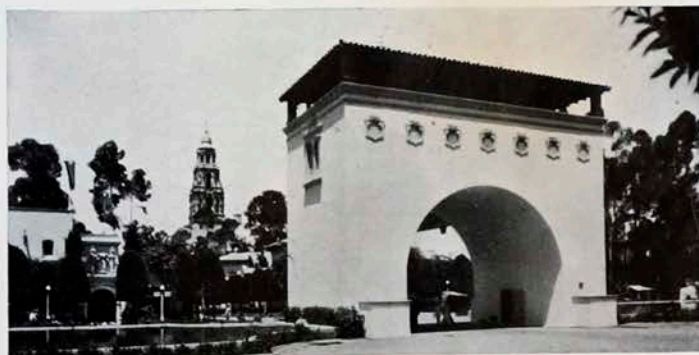
The Arch Way
