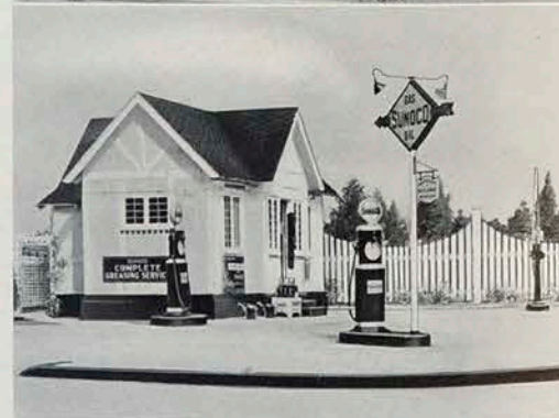
Even the gas station modernizes. Small projects like this are well worth "before and after" photographs. Photograph from Federal Housing Administration.
