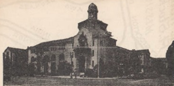
HEADQUARTERS BUILDING: 2601 SOUTH FIGUEROA STREET, LOS ANGELES
