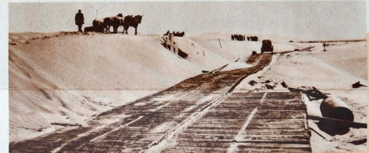
YUMA ROAD, U. S. A.—This highway, first built of plank laid on desert sand, is reproduced as a part of the Ford roadway exhibit. The Yuma Road runs from El Centro, California, to Yuma, Arizona. It now is a modern, paved highway. It crosses desert country that is beautiful and picturesque and accommodates much traffic the year 'round.
