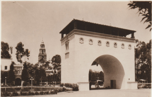
The Arch Way
